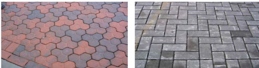
A. Examples of types of block pavers used in permeable paving systems
